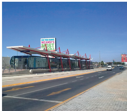
BRT station in Soweto showing the potential for local economic development.
